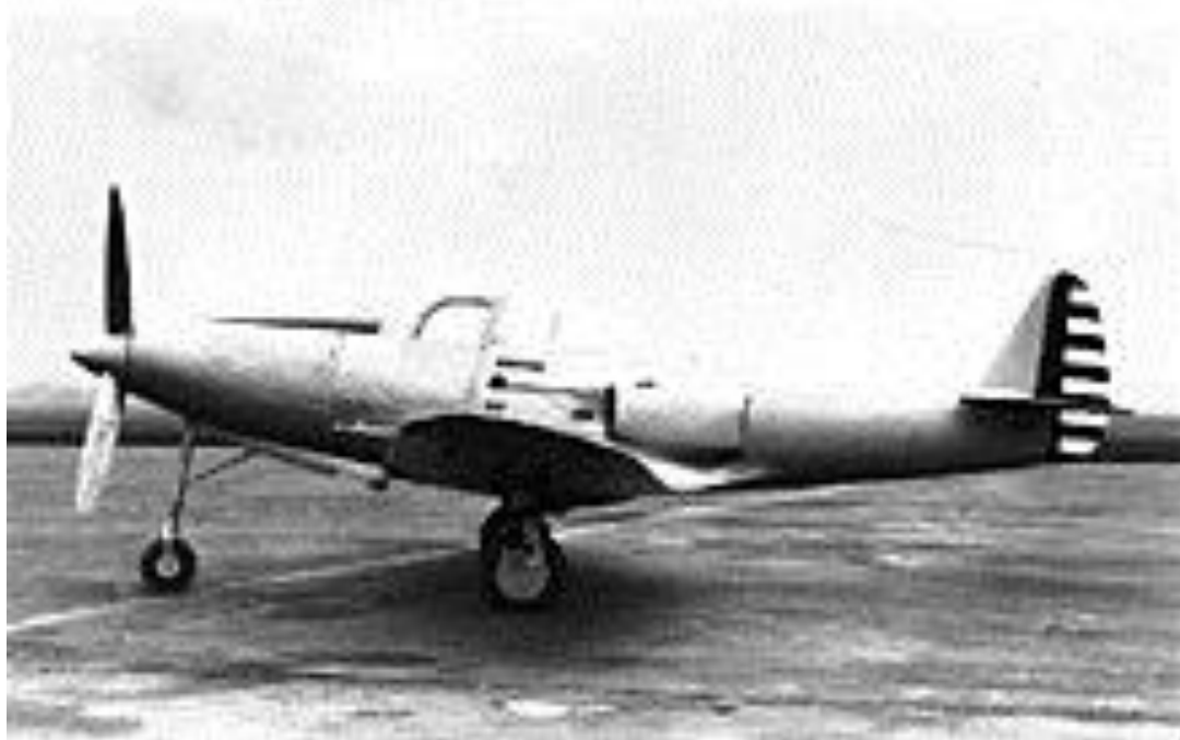
Bell XP-39 showing the position of the supercharger air intake
