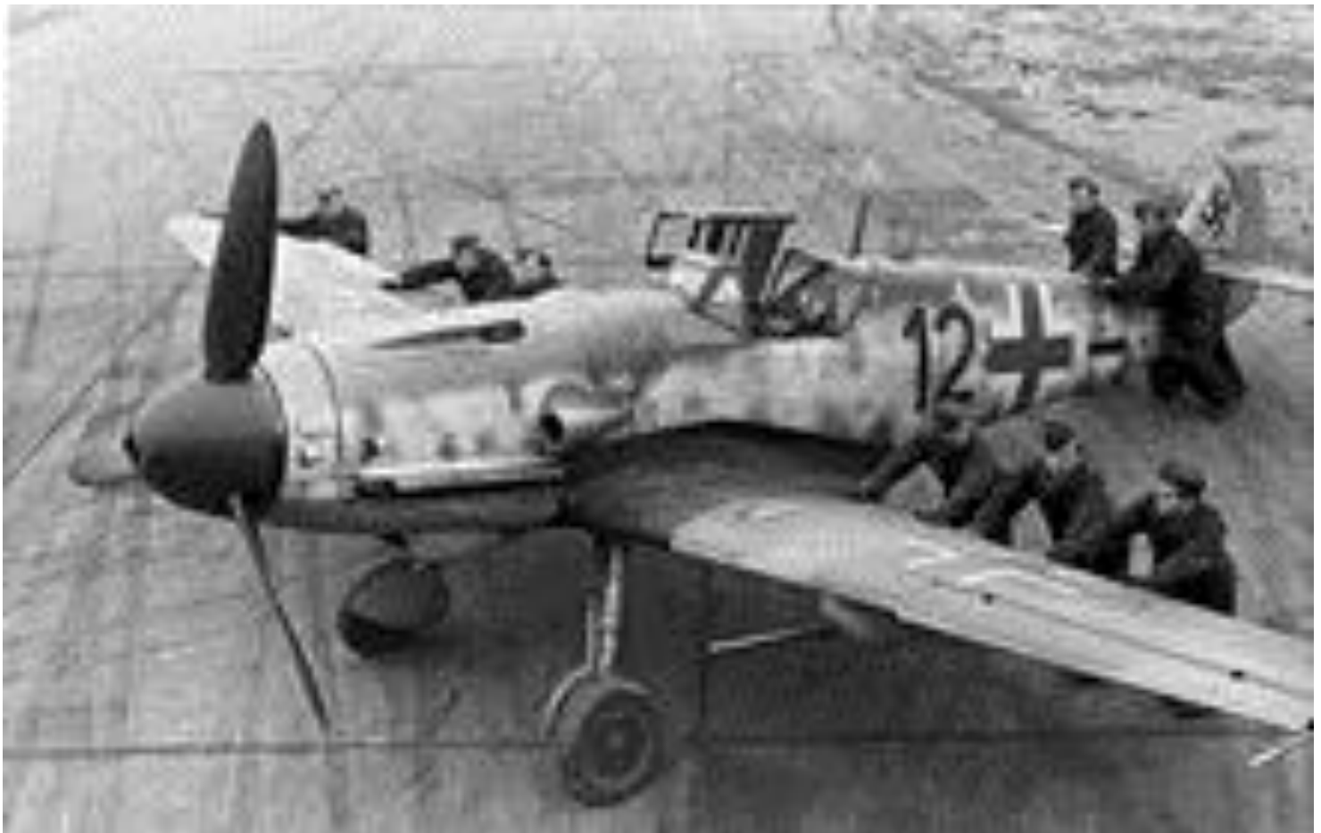
Luftwaffe ground-crew positioning a Bf 109G-6 equipped with the Rüstsatz VI underwing gondola cannon kit. Note the slat on the leading edge of the port wing. JG 2 , France, late 1943.
