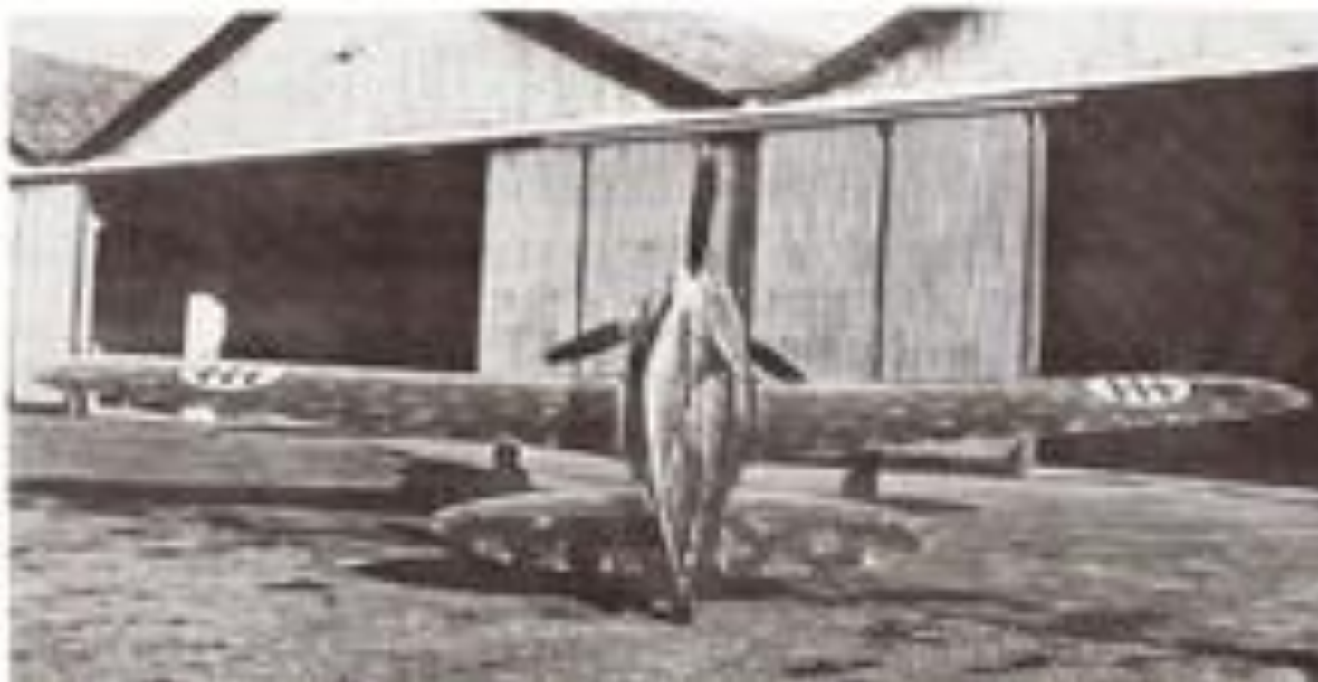
Revised and camouflaged C.202 prototype from the rear, showing the three-bladed propeller and wing profile
