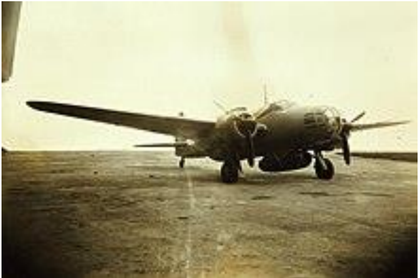
A modified Ki-48 with a Ne-0 turbojet under the bomb bay during testing
