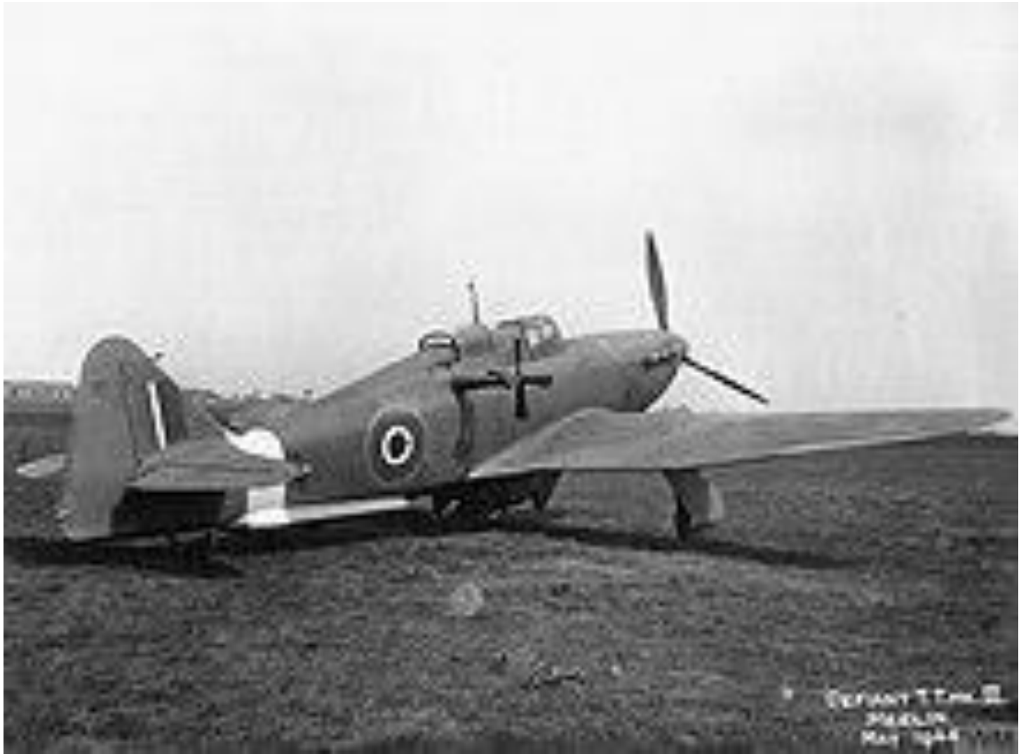
Defiant TT Mk III target tug, number N1697 ; RAF Desford , May 1944. The wind-driven generator provided power for the target winch
