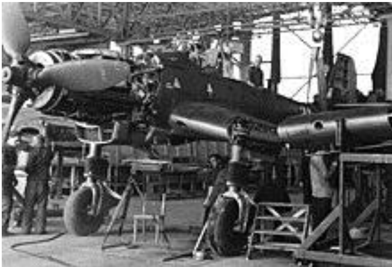
A Ju 87D during wing installation
